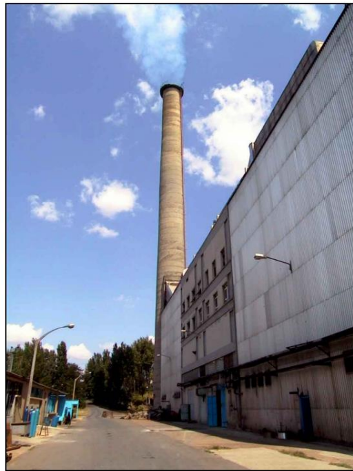
Figure 4: Stack for Units 4 and at Ambarli Fuel Oil Plant
